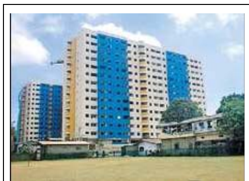
Figure 6.1 Sahaspura housing project Source-Sustainable Township Program
